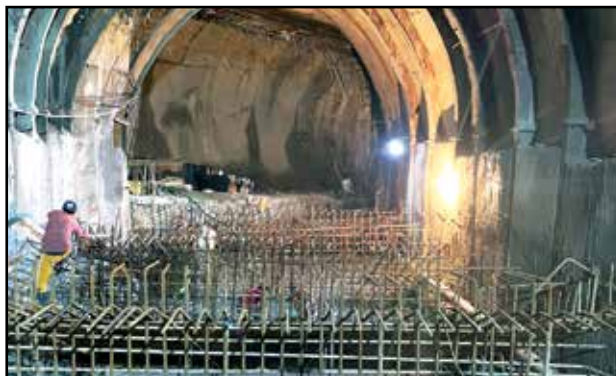
Adit Junction Head Race Tunnel
