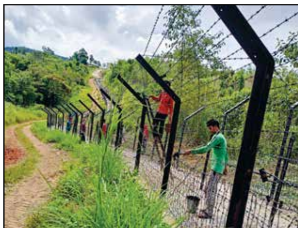
Fencing Work in Progress, Tripura
