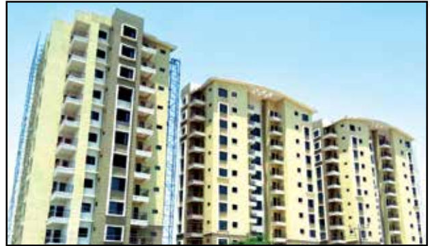
G+11 Jammu Development Authority Flats, Muthi
