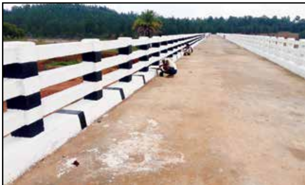
PMGSY Bridge works Gumla district
