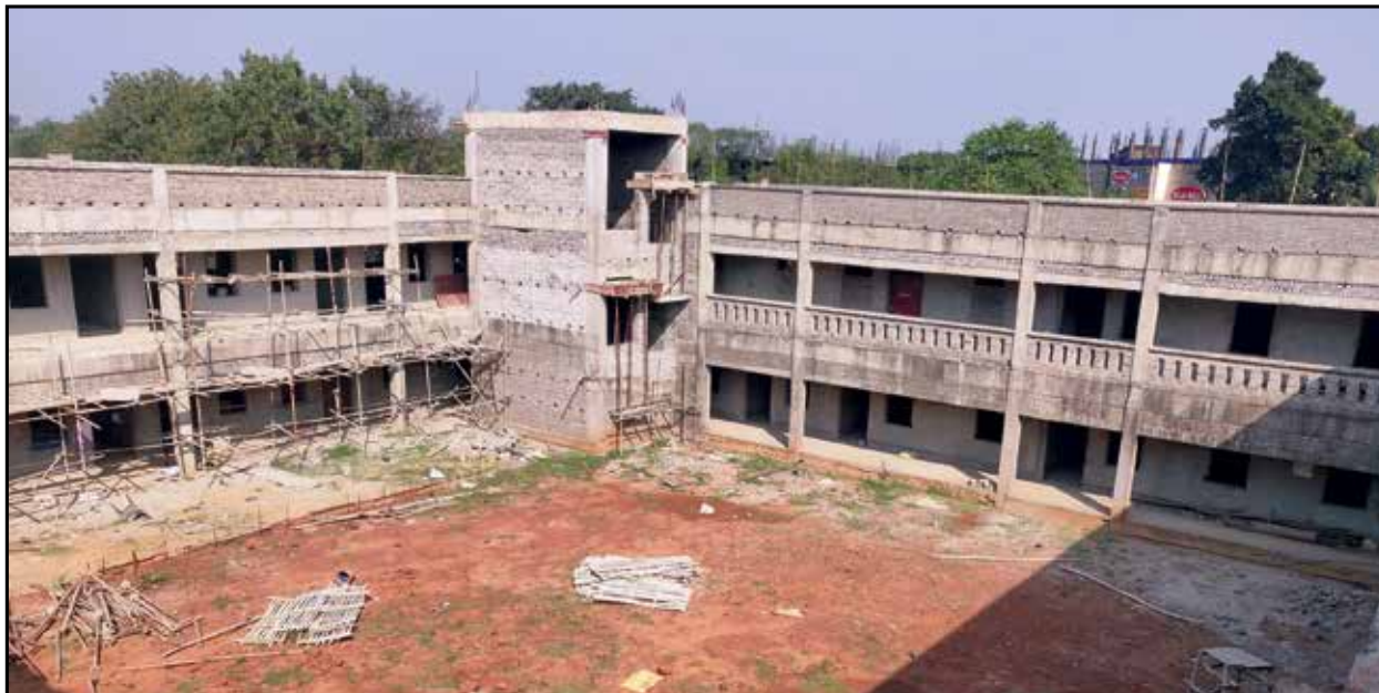
Construction of School Building at KVS, Kharagpur
