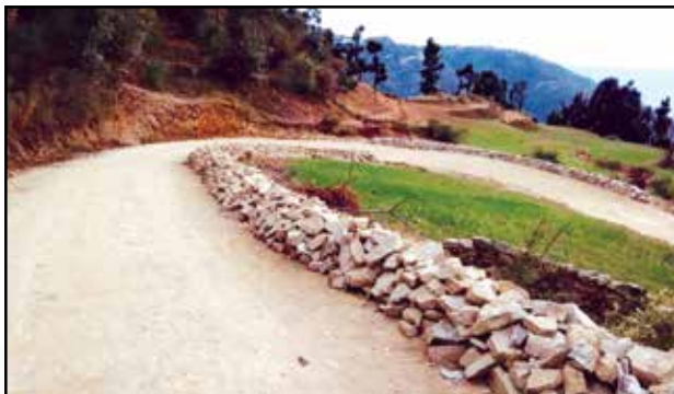
Road Works in Progress
