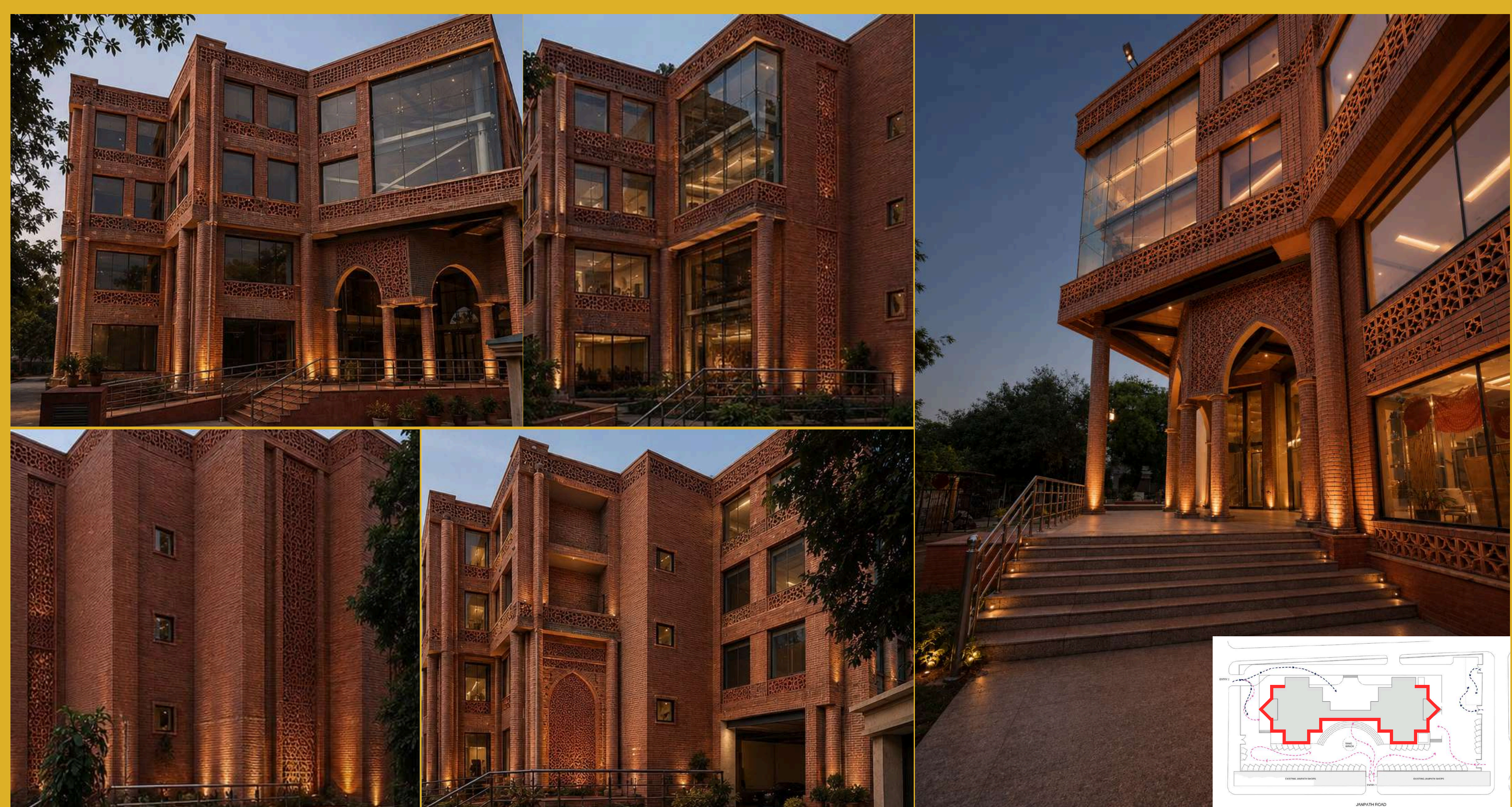
BRICK CLADDING COMBINED WITH TERRACOTTA JALI ON MS FRAME
