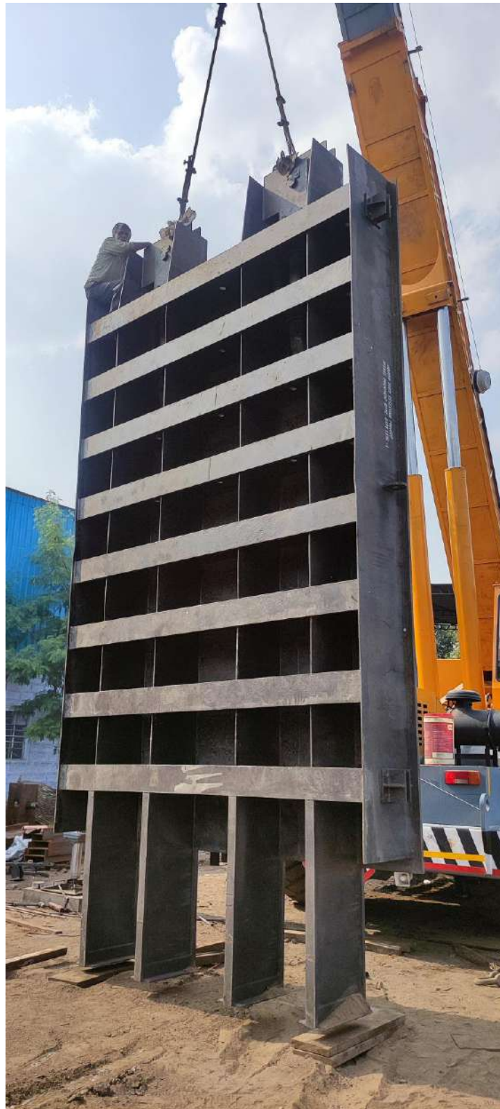
(E) Intake Bulk Head (2.67 m x 4.59 m)
