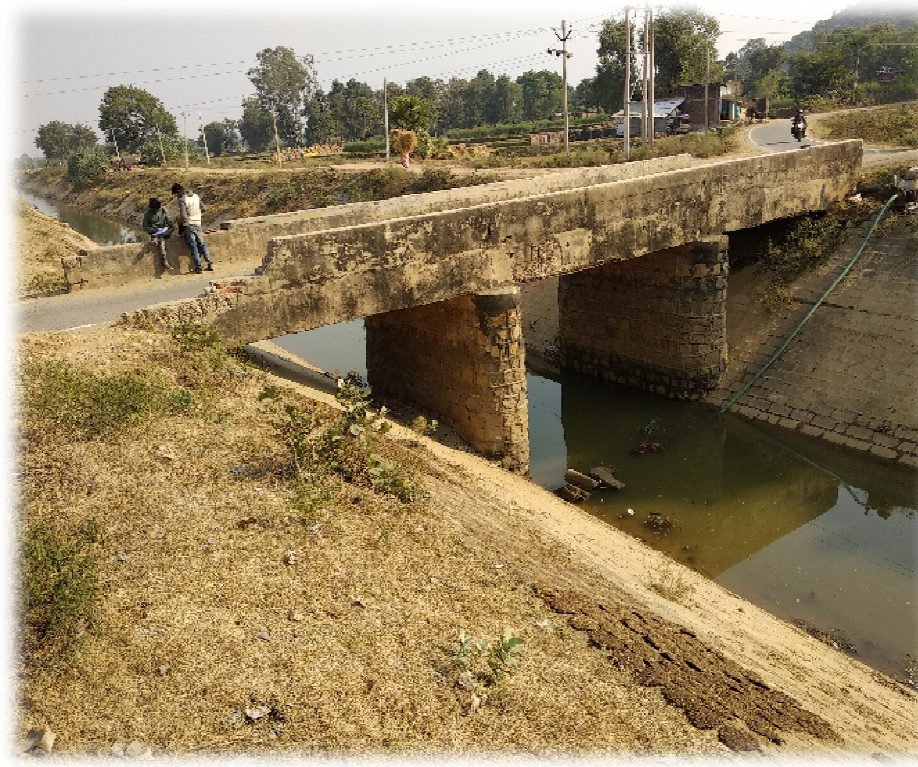
S.L.R BRIDGE AT CH. 69.525 KM
