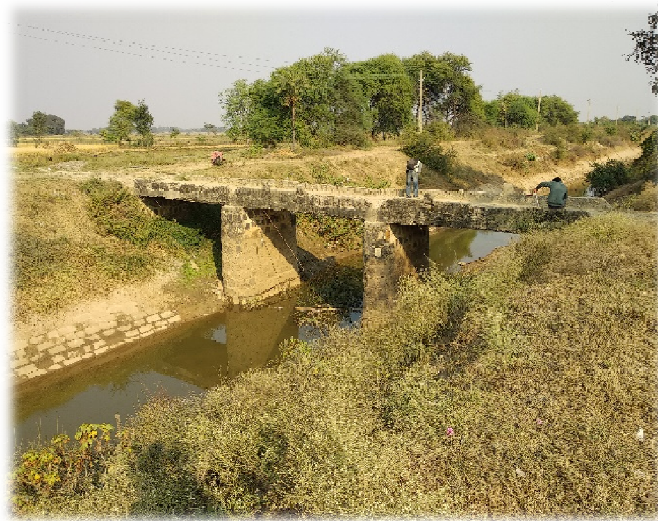
CART BRIDGE AT CH. 68.671 KM
