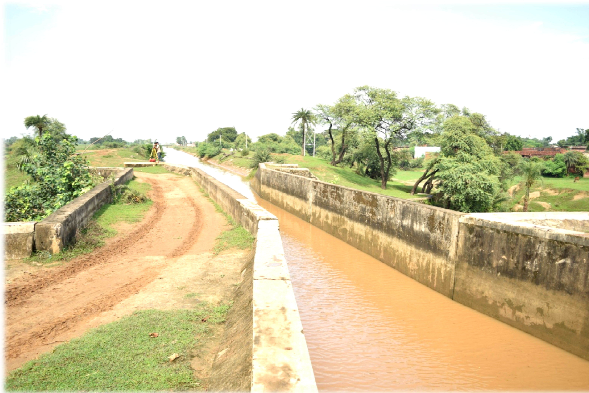
RD 71.02 SYPHON AQUEDUCT OVER TEKARI RIVER
