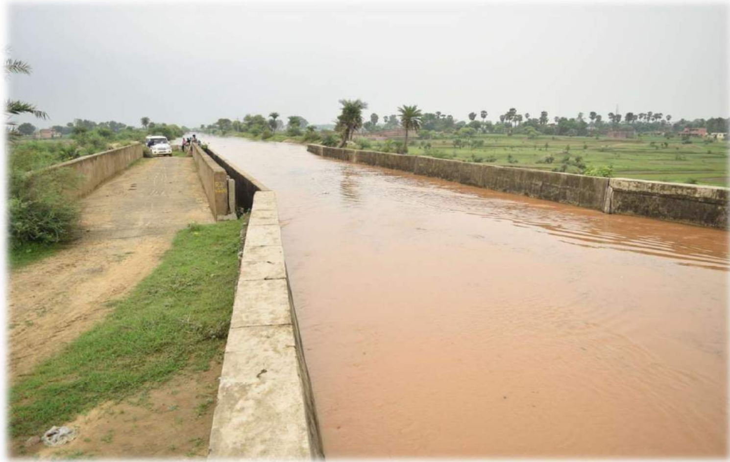
RD 14.39 AQUEDUCT OVER NALLA
