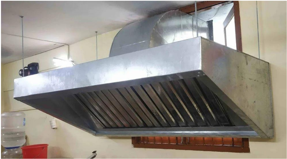
SS HOOD WITH SS FILTER 304 GRADE OF SIZE 36X30X24
