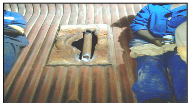
Damaged Water Wall Tubes
