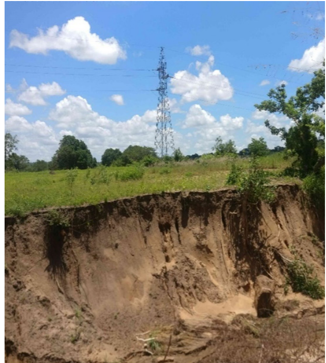
Soil Erosion due to flowing river near critical tower locations
