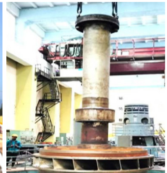
Lifting/Dismantling of Runner with Turbine shaft of Unit-04 completed
