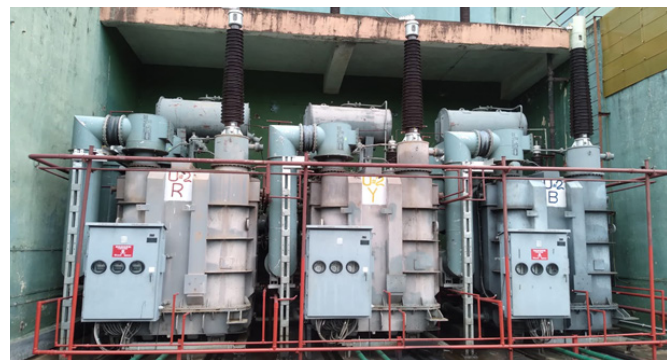
23.4 MVA Generator Transformer (GT): Unit-02: Three (3) Nos. new installed
