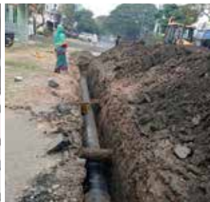
Excavation and laying work of distribution mains pipe line DI K9 in progress -Nandanwan 2, Zone -05
