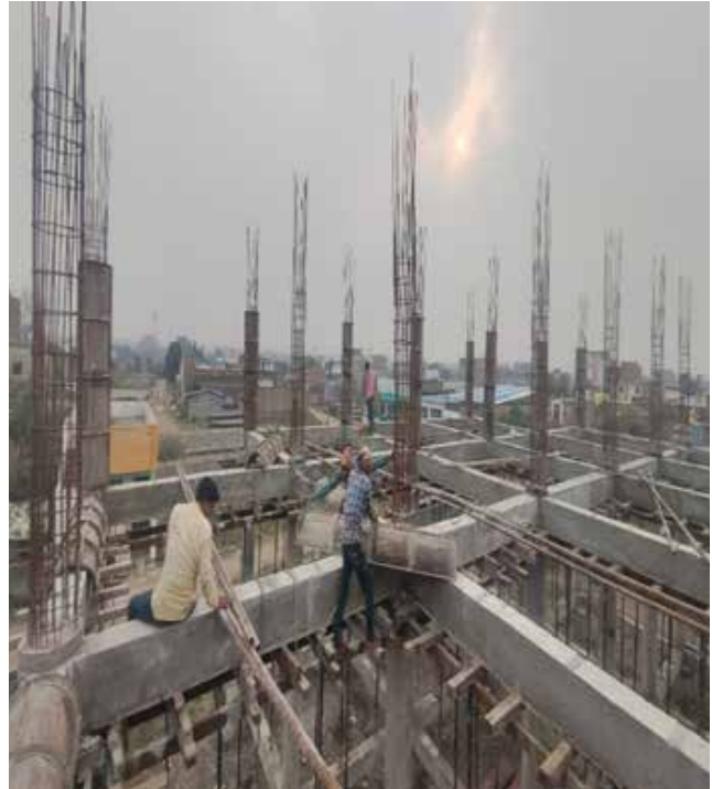
Steel binding of 1st Lift Column above 1st brace beam in progress at Kalamna Wanjara ESR, Zone-08
