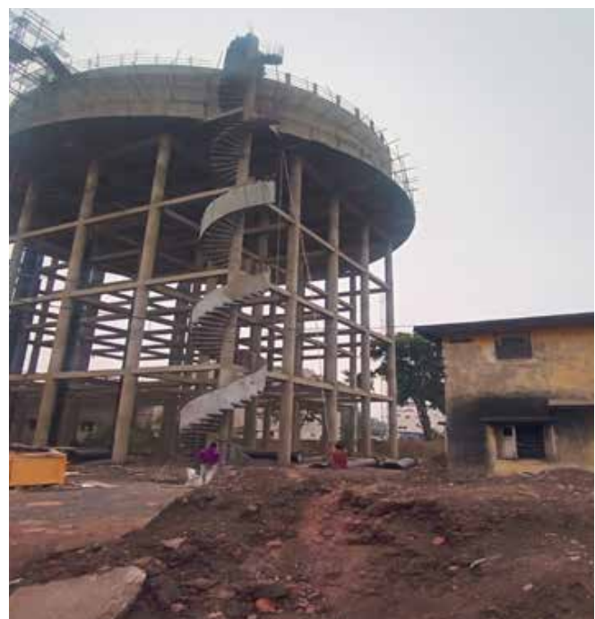
Compound Wall & Staircase pardi steel binding work in progress at Nalanda Nagar-1 ESR, Zone-3
