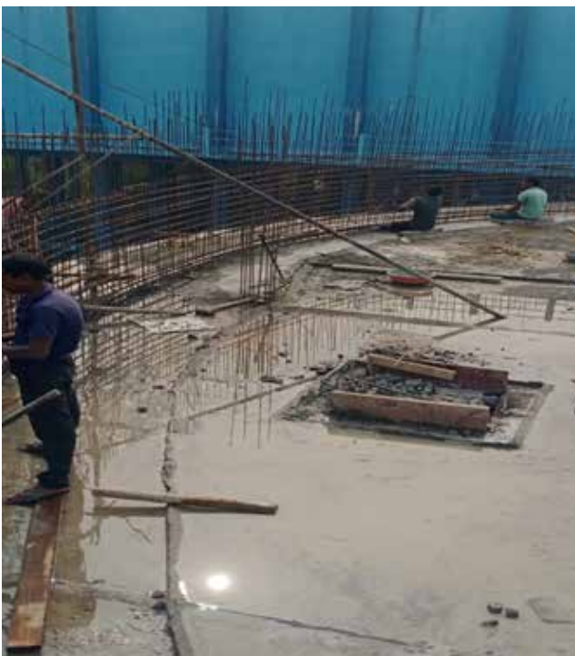
Steel binding work of 1st lift container wall in progress at Nari-1 ESR, Zone- 09
