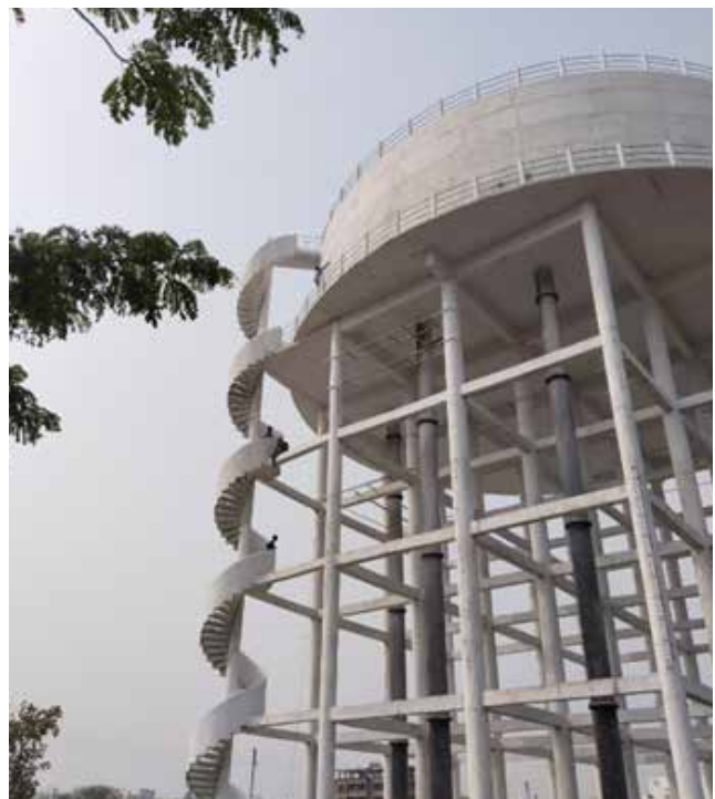
Painting & Grouting Works in progress at Dabha 1 ESR, Zone-02
