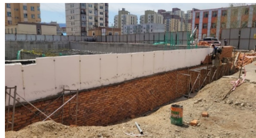
Brick Masonry Work (120 mm thick above 100 mm XPS Insulation)
