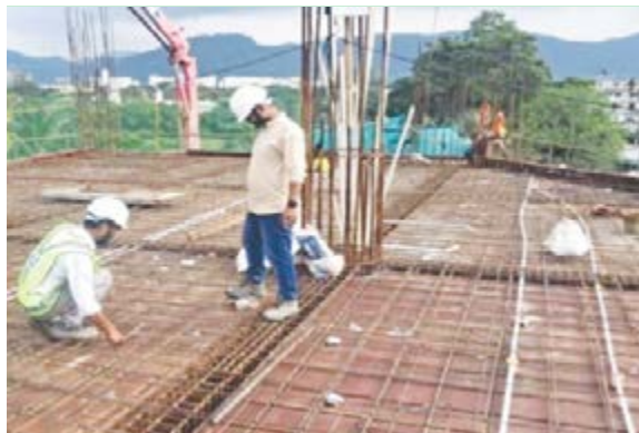
Auditorium Column Shuttering & steel tying work in progress
