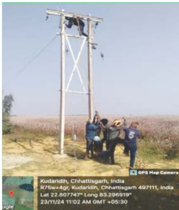
Double Pole of Erection work (11 kV line)
