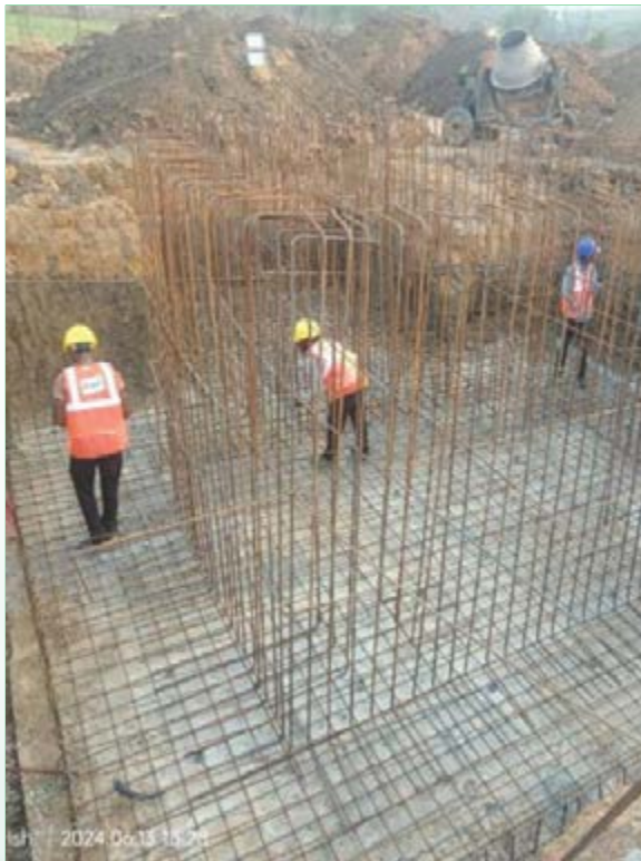
Foundation of Power Transformer
