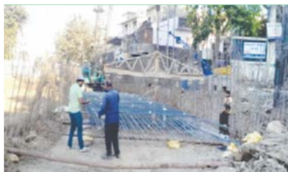
Diaphragm Wall work in progress
