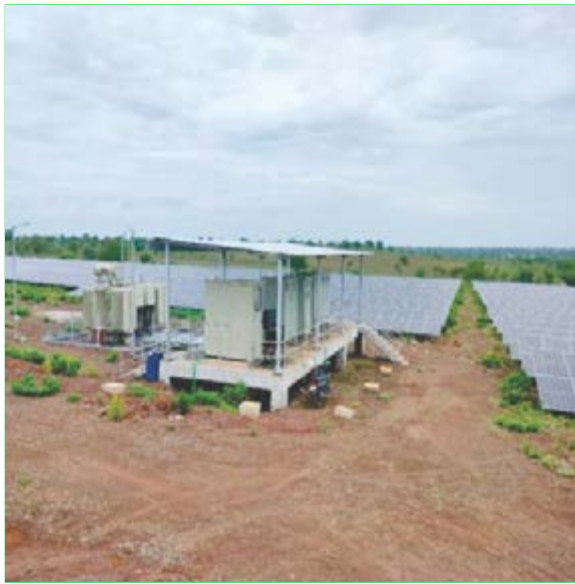
Solar Panel & IDT installed at site
