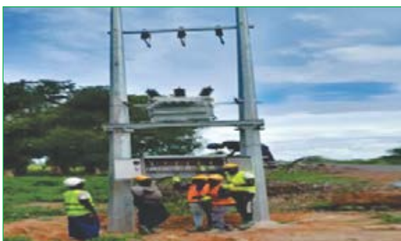
Installation of MV Poles
