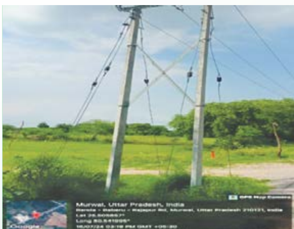
Double Pole erection works
