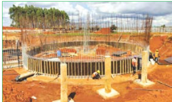
Clariflocculator B outer wall shuttering work in progress-Njombe WTP
