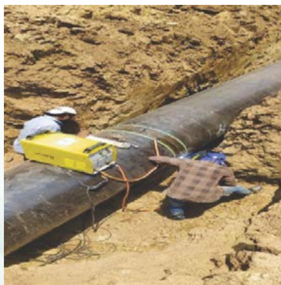
Welding of M.S. Pipe in progress
