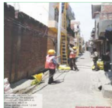
AB Cable erection works
