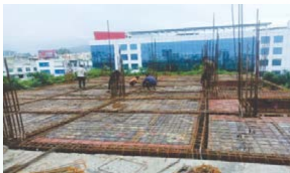
Reinforcement work in progress at site
