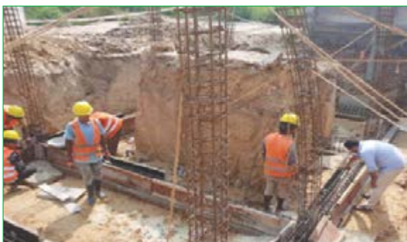
Formworks and R.C.C works for guard house lower tie beam at Khajura, Banke
