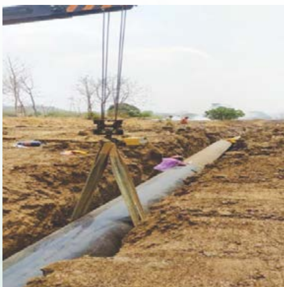
M.S. Pipe Laying Work in progress
