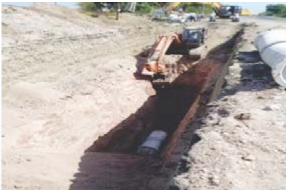
RCC NP 4 Pipeline laying work
