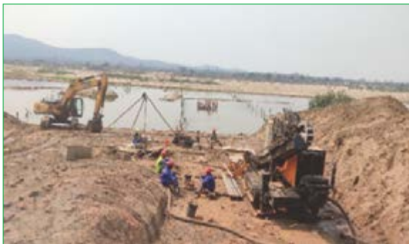
River crossing by HDD method on Robuvue River
