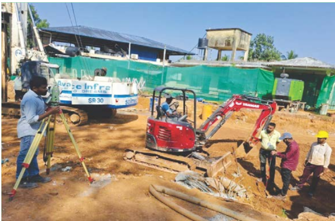
Setting Out of Pile Layout
