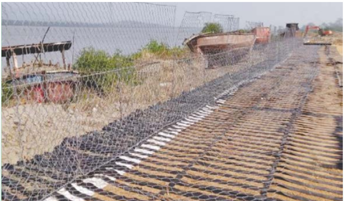
Gabion box & Paralink fixed at Naglabunder site
