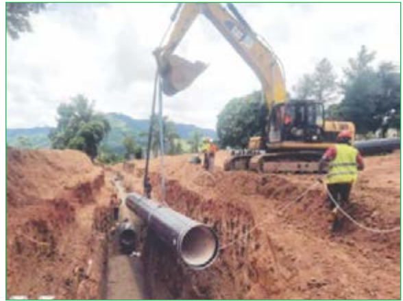
Laying of 914mm Water Pipeline
