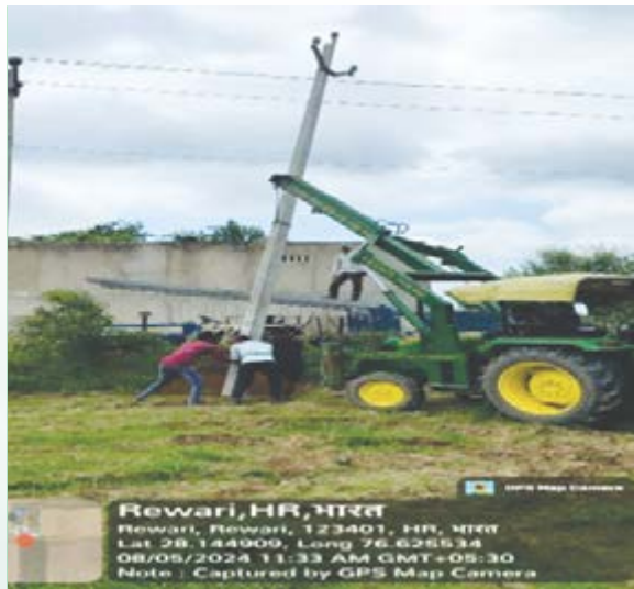
Pole erection works
