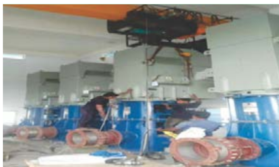
V.T. Pump Installation at Tappar Dam based Water Supply Project
