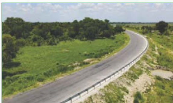
Metal Beam Crash Barrier work completed at Km 27+000
