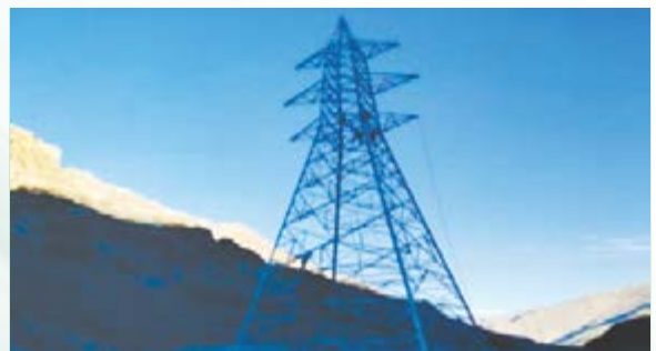
Erected DB type Tower for Transmission Line - 66 kV (Dah - Hanu - Khalstse)
