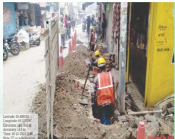
Underground Cabling work excavation in progress
