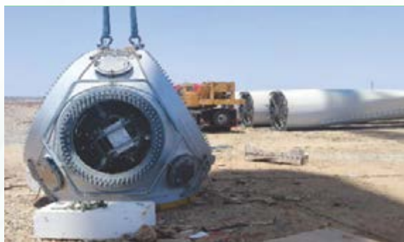
WTG Hub under erection at site
