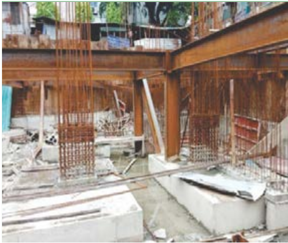
Column 1st Lift (Zone-I) Reinforcement work in progress at site
