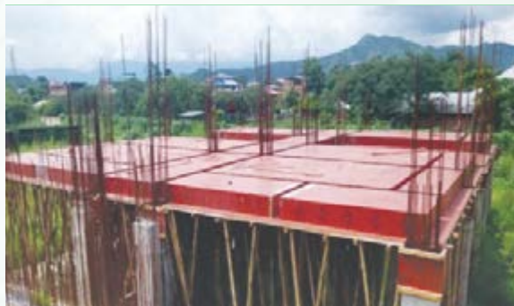
Roof Slab shuttering for Block-B
