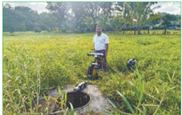
CCTV inspection for Wastewater Pipes
