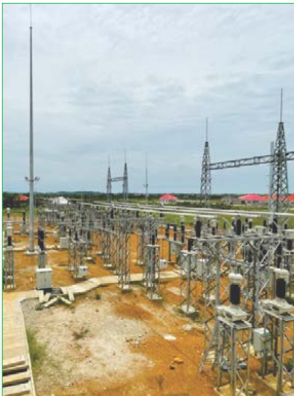
66/22kV & 66/33kV Switch yard PCC and 66kV Multi Circuit erection
