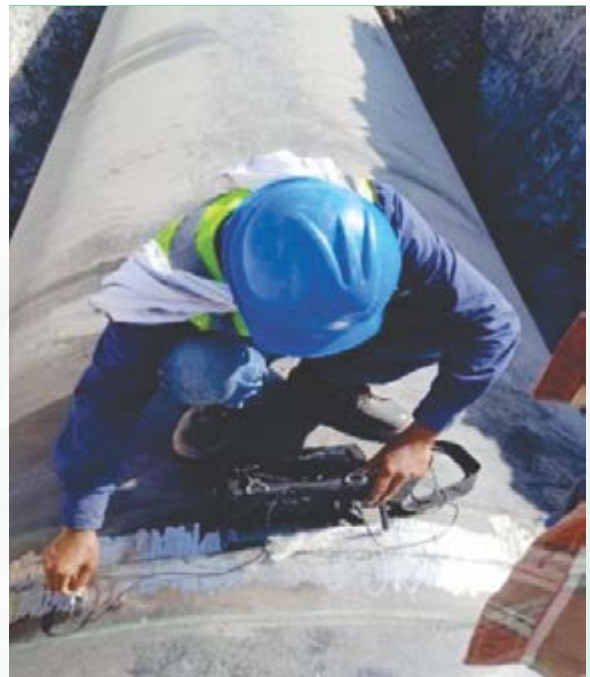
U.T. Performing at site of Budhel to Borda Bulk Pipeline Project
