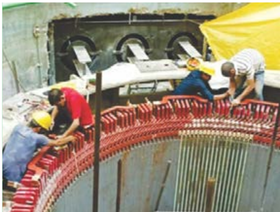
Jumpering of wound stator (top & bottom bar) of top side of Unit No. 3
