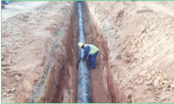
Pipeline Laying on T3 line in Matema
