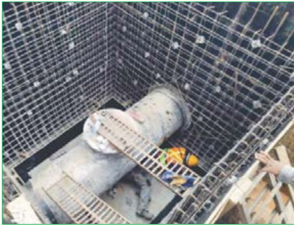
Construction of Air-valve chamber
