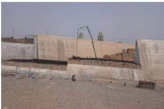
Concreting work in progress in D/S Guide Wall
