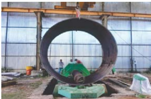
Pressure Shaft Liner is under fabrication at Site
