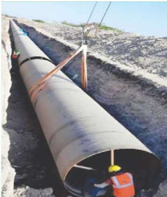
2000mm dia M.S. Pipe laying work under progress at Navada
