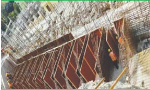
400 kV New Khimti RCC Counter forte retaining wall Bar binding & Shuttering work
