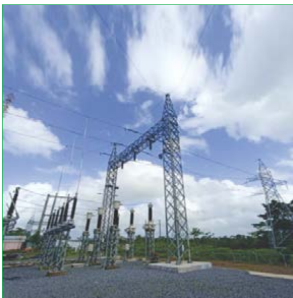
Gantry Connection between 138 kV single circuit line and La Esperanza Substation
