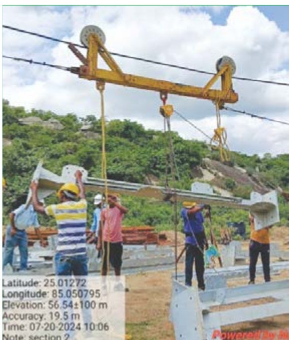
Shifting of materials through Material Ropeway Vanabar Ropeway, Jehanabad
