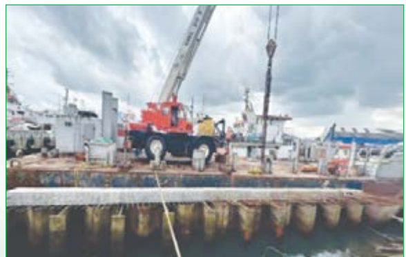
Installation of Precast Concrete Panels
