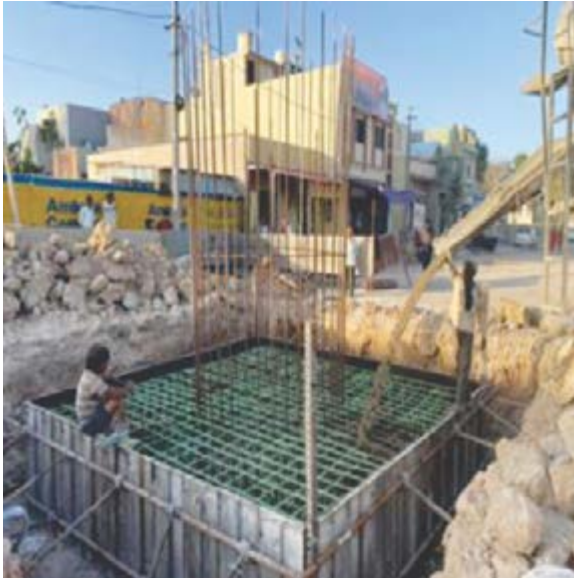
Pile CAP concreting work
