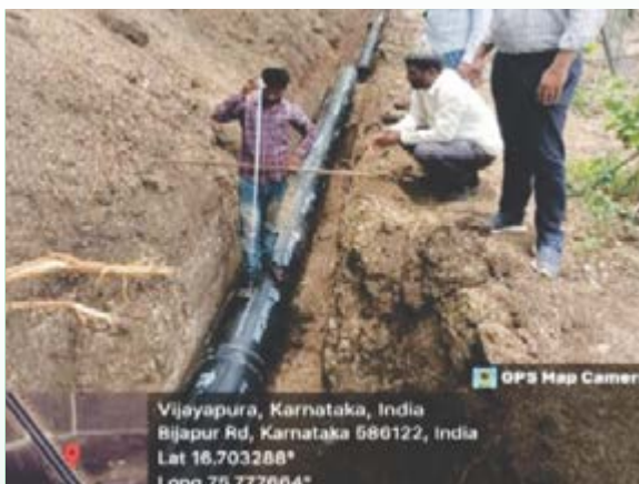
Zone-37 Bulk Main MS pipe of dia 400mm BMP-103 from BMJ-33 to BMJ-15 excavation trench
