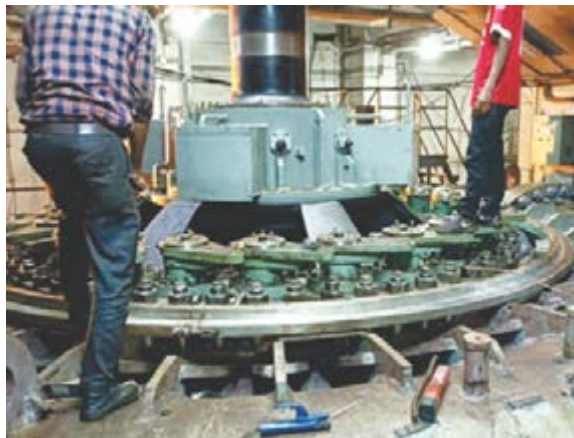
Trial Assembly of Guide Apparatus of Unit No. 4
