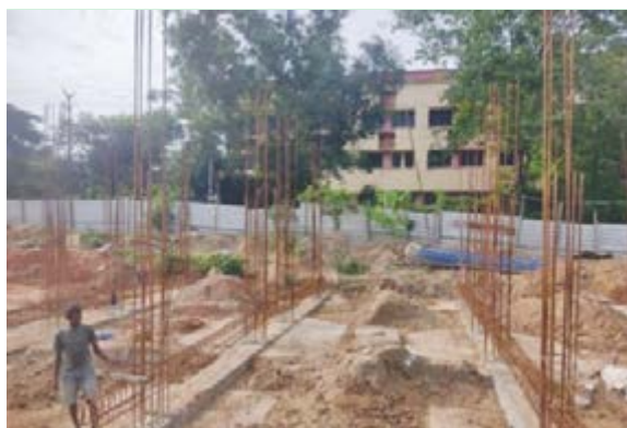
Plinth beam reinforcement work at site
