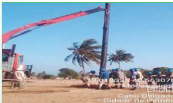
MV pole erection at Chuiba
