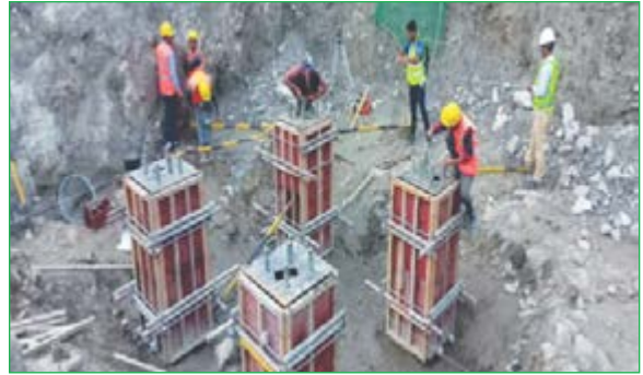
400 kV Barhabise S/Stn. T1 Tower Foundation bolt fixing
