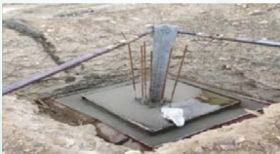
Ongoing foundation works for Transmission Line - 66 kV (Dah - Hanu - Khalstse)
