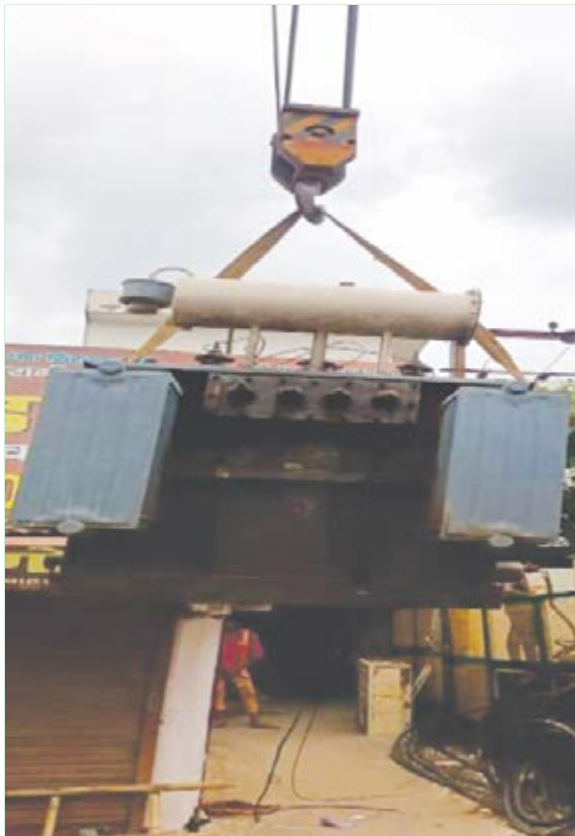
Dismantling of transformer
