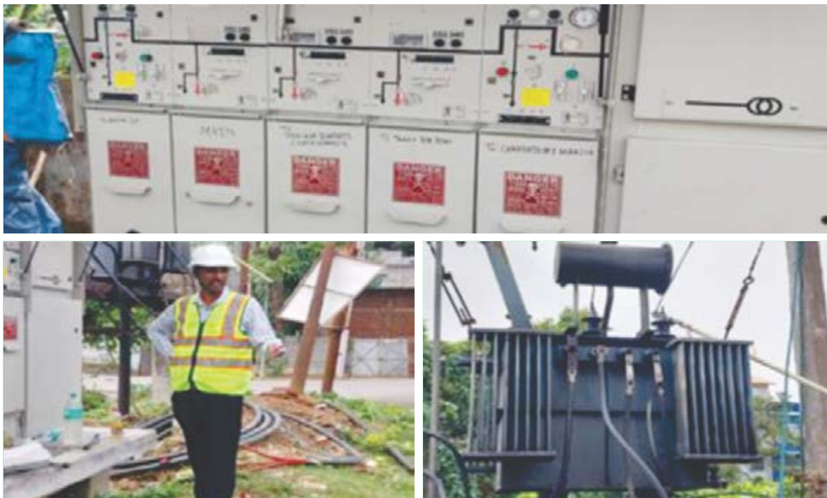
11kV RMU commissioning works for Dhaleswar, Shivmandir feeder
