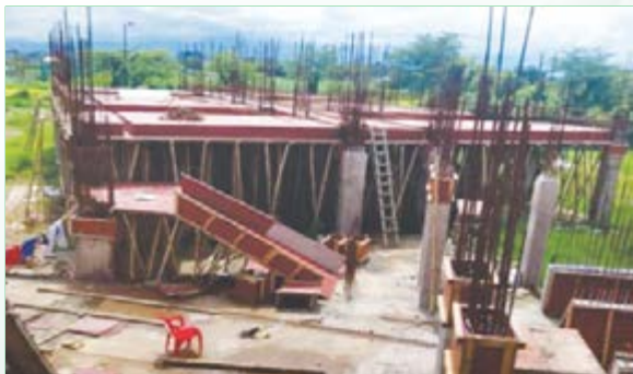
Roof Slab and Column Casting of Block-A
