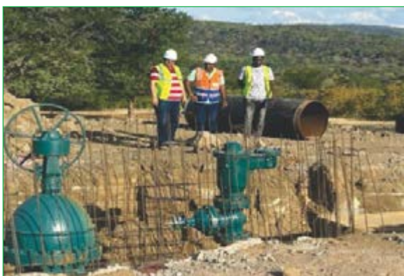
Installation of valves at site
