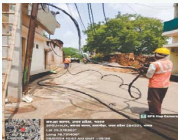
AB Cable erection works
