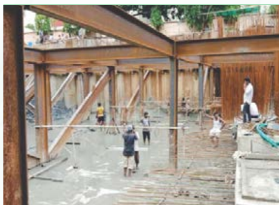
Basement Raft (Zone-II) Reinforcement work in progress at site
