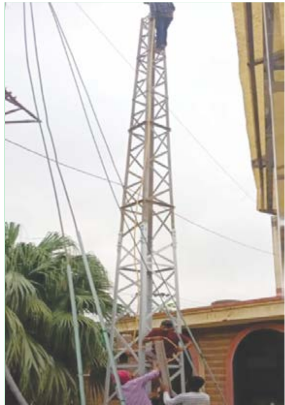
Erection of Lattice Tower
