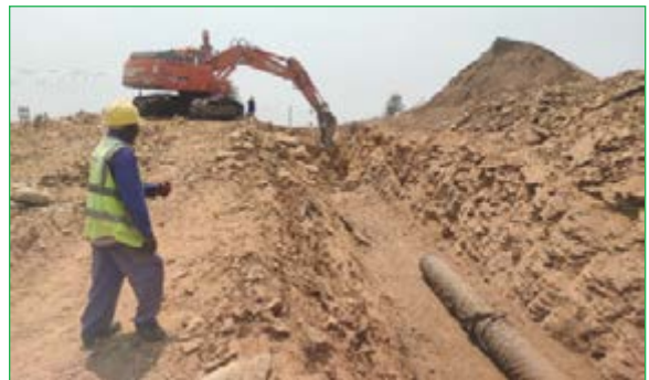
Pipe Laying Over Mountain on Transmission line T4 to Moatize
