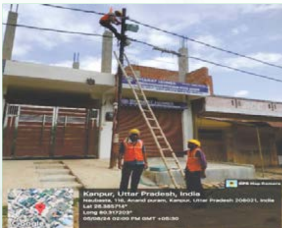
Replacement of bare conductors/ Damage cable with AB cables
