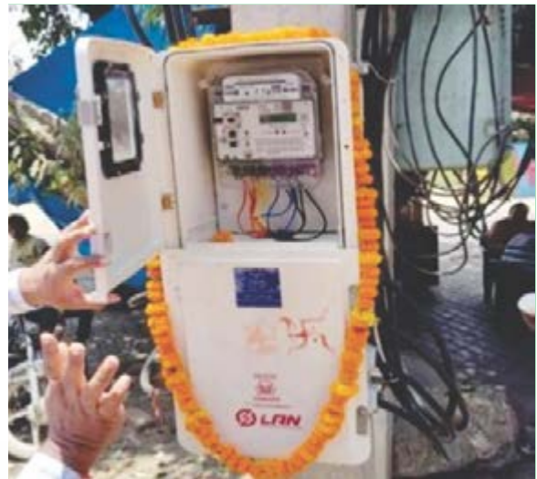
Installation of DT Meter
