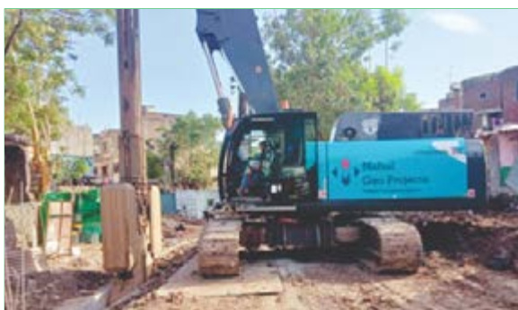
Diaphragm Wall excavation work in progress
