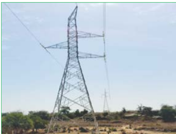
Single Circuit Transmission Line
