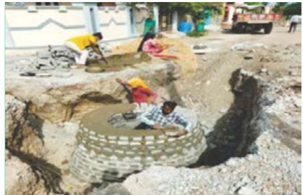
Construction of Manhole
