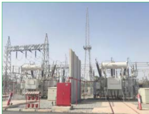
2 Nos. of 25MVA Power Transformers at Mango Substation
