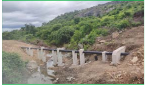
Pipe Carrying Bridge over stream on Transmission line (T4) in Moatize
