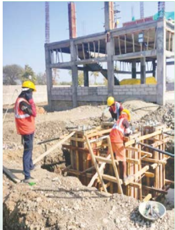
Foundation of tower of switchyard
