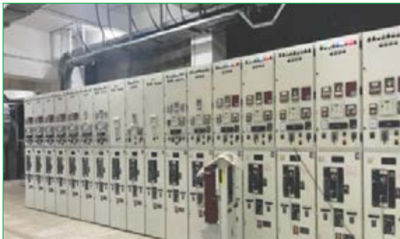
Charged HT Station Auxiliary Board-I (SAB) at Switch Gear Room
