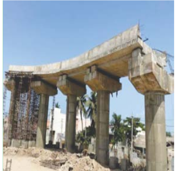
Deck Slab casting work
