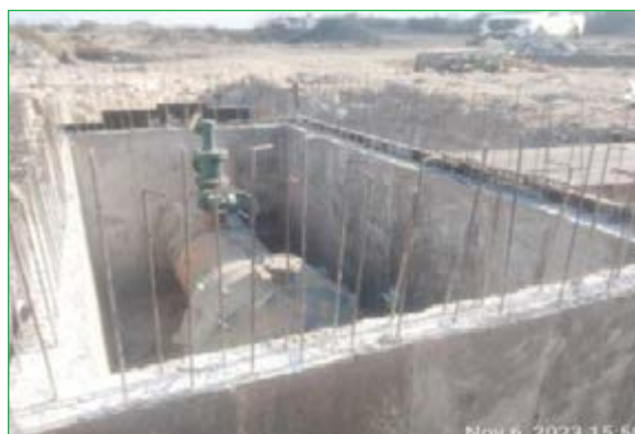
Construction of zero velocity valve chambers
