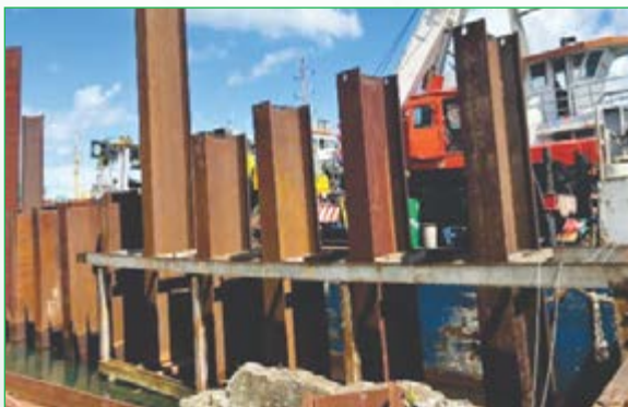
Installation of King pile and Sheet Pile
