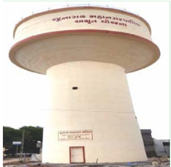
Elevated Service Reservoir of 13 Lakh Liter Capacity
