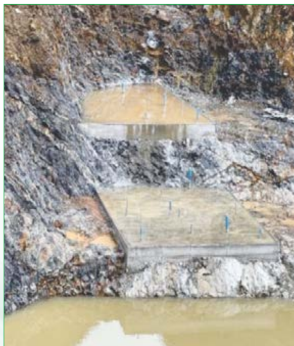
Dam Foundation Levelling PCC
