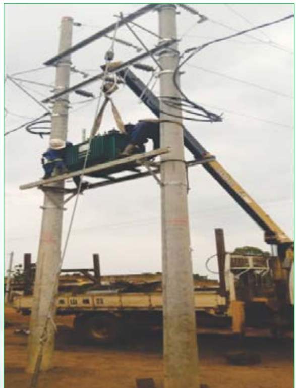
Installation of Transformer
