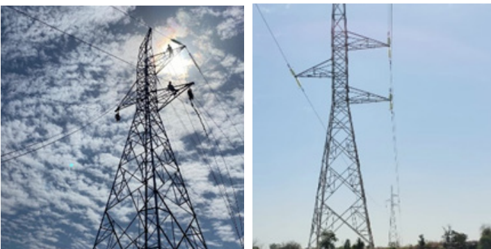
Stringing works in progress - Dapaong-Mango Transmission Line
