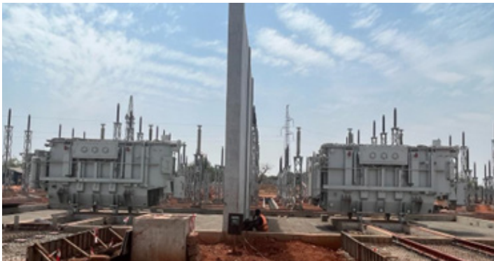
Dapaong Substation: 2Nos. of 25MVA Power Transformer Installed
