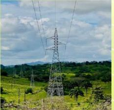
138 Kv Single Circuit Transmission Line Stringing Completed
