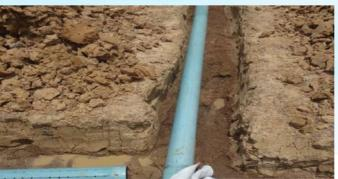
Excavation of trenches and laying of PVC pipes in d/s of Kpong Dam
