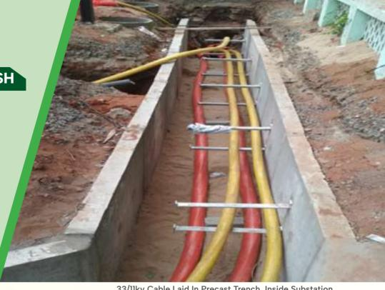
33/11kv Cable Laid In Precast Trench Inside Substation
