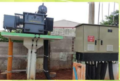
11/0.4 Kv Distribution Transformer With Lt Feeder Pillar Box
