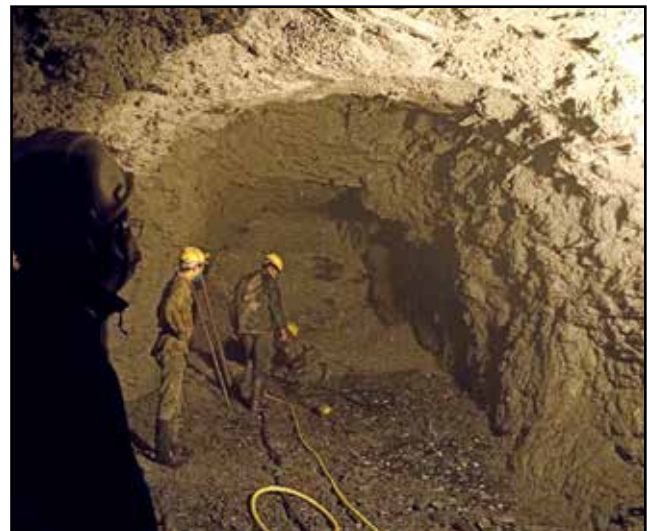
Excavation of Head Race Tunnel (HRT) and Pressure Shaft (PS) in progress
