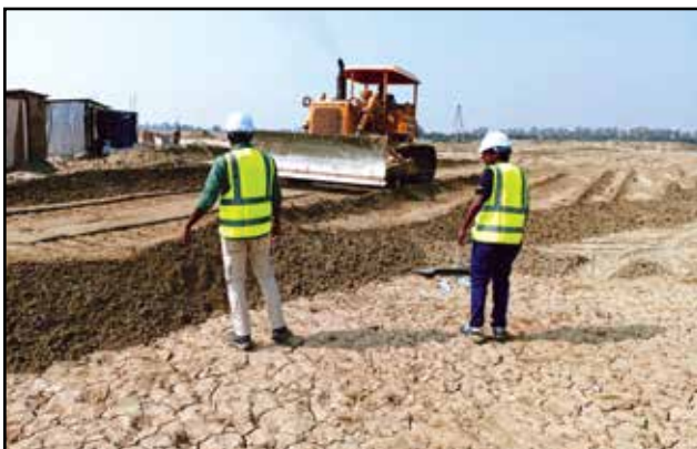
Land filling at 400/132kV GIS Rahanpur Substation
