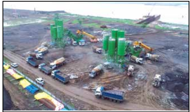
Right Bank Cofferdam and Batching Plant
