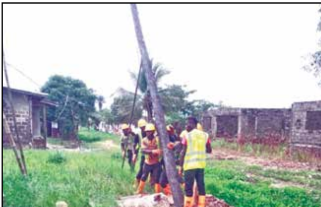
Erection of Wooden Poles at Site
