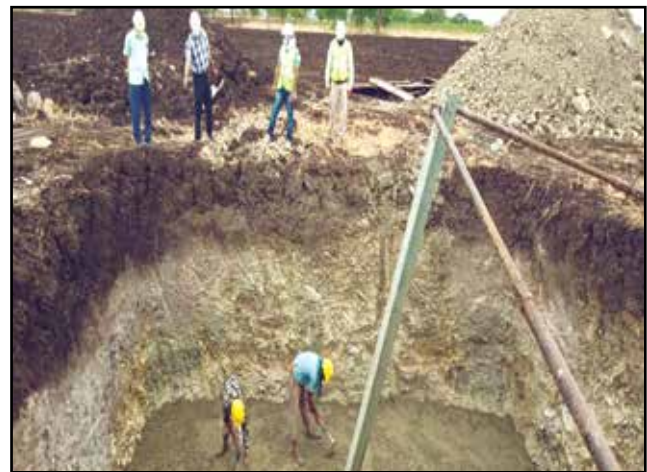
Tower Foundation works in progress at 220 kV Kanwan - Dhar Transmission Line
