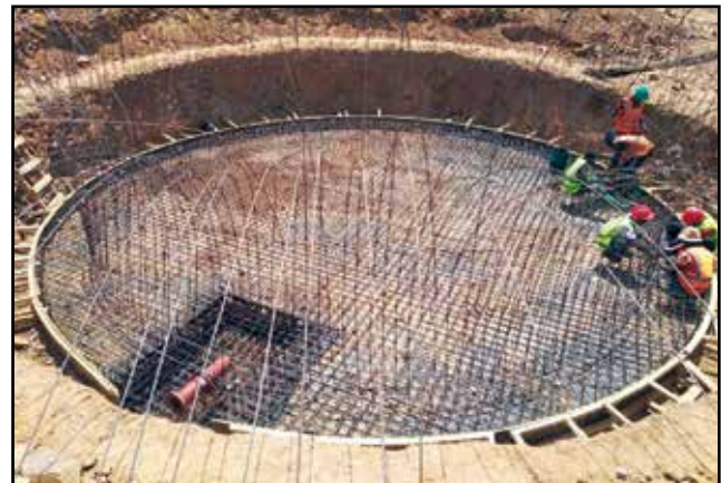
Reinforcement Binding of Foundation Raft of Mgela Tank- Ground Level Service Reservoir
