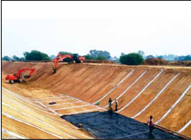
Lining in Progress at Right Main Canal
