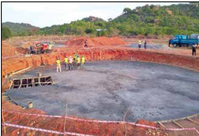
Buchama Tank Plain Cement Concrete
