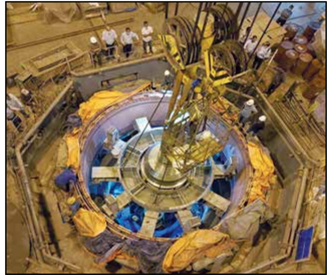
Unit 6 after lowering of Generator shaft along with LCB
