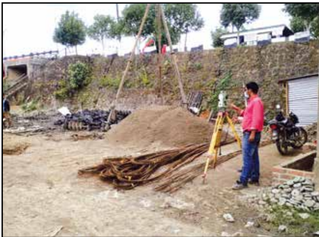
Pile point layout marking at 0.45 ML Over Head Tank at Old Thumbuthong
