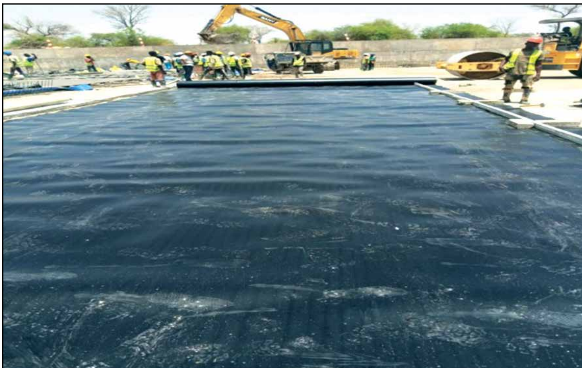
Laying of Geo Membrane
