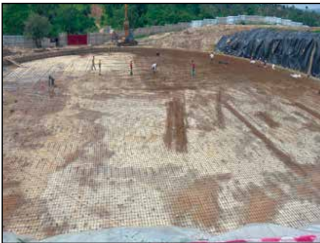
Raft Reinforcement at Kibamba Reservoir (10 MLD)
