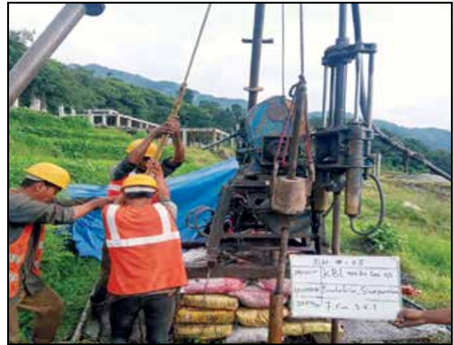
Soil Investigation work in progress at 400/220kV New Khimti GIS Substation site
