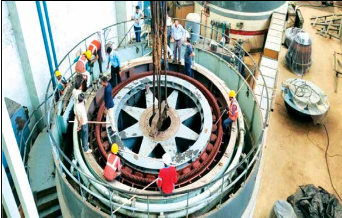
Assembly works (Placing Rotor in the pit)
