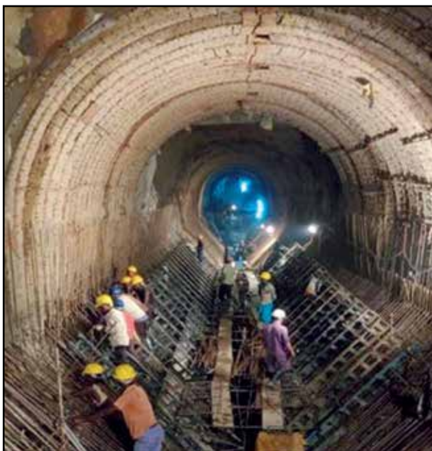
Concrete lining of Desilting of Basin in progress
