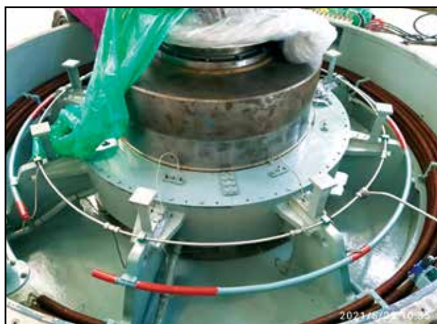
Rectification work for Arresting Oil Leakage of upper Combined Bearing House
