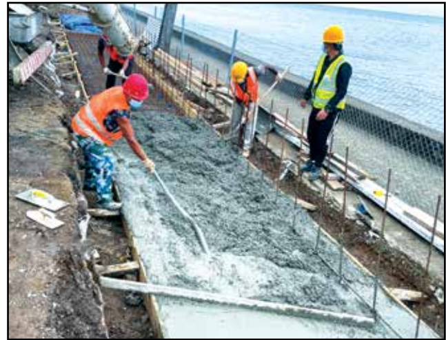
Construction of Retaining wall to Support the Road Embankment along Area 1
