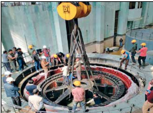
Rotor Lifting of Unit-1 Generator from pit
