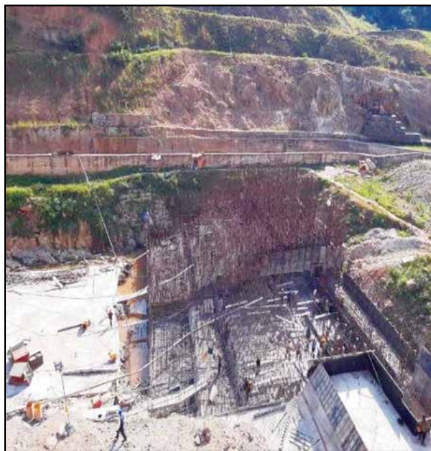
Concreting of dam left bank blocks
