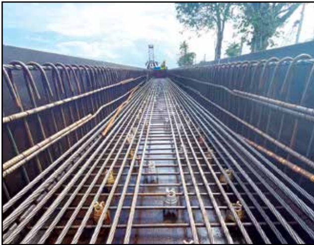
Pre-stress Beam reinforcement tying works in progress for Nasese Bridge
