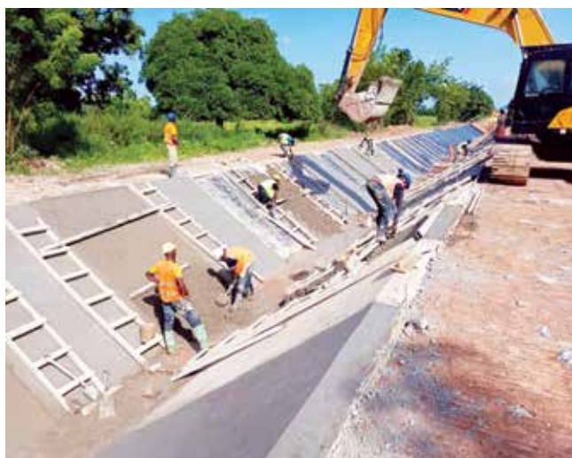
Construction (concrete lining) of Left Bank Canal
