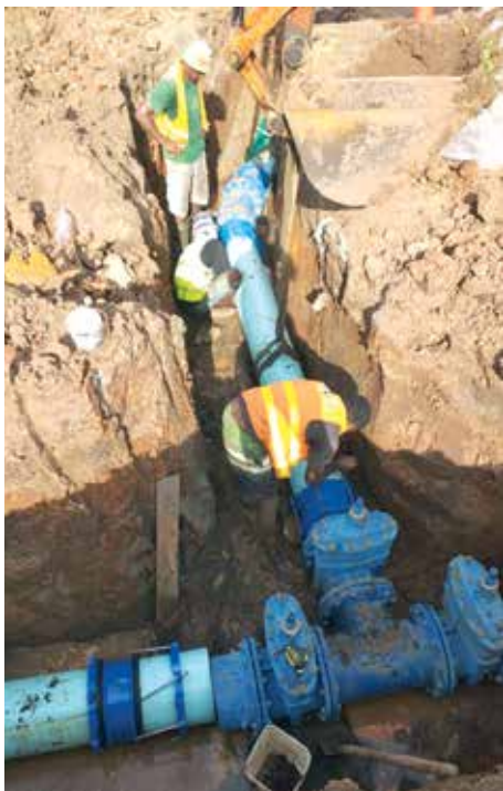
T Connection of pipelines
