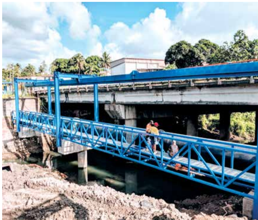
Commissioned 4 Mile Bridge sewer pipeline
