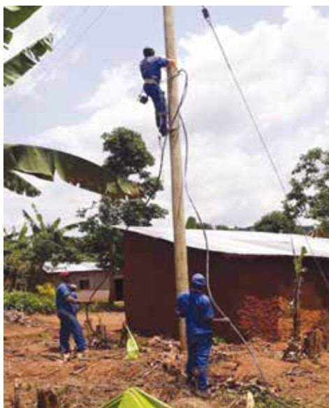
Stringing of AB Cable for the project Supervision of Rural Electrification Projects in Rwamagana, Kayonza, Ngoma and Kirehe Districts
