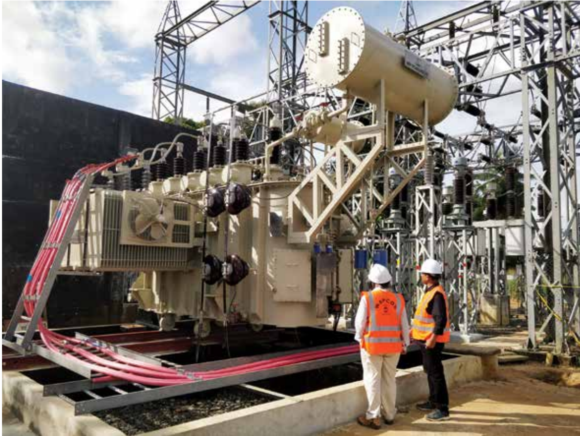
Final check of Commissioned Transformer by WAPCOS Experts at Paynesville Substation for the project "Consultancy Services for the construction of the 66/33/22kV transmission and Distribution network in Monrovia and Bomi/Grand Cape Mount Countries" in Liberia.
