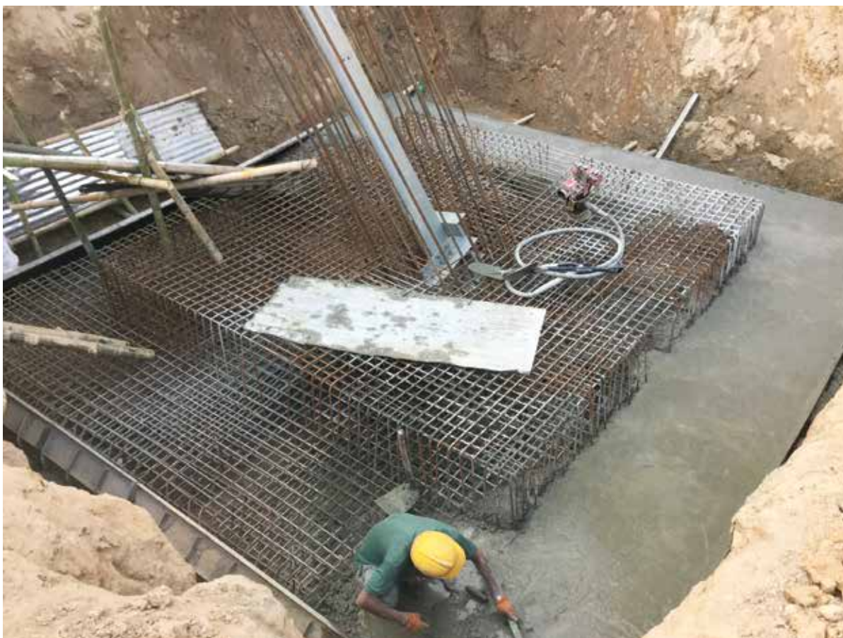
Pouring of M-20 concrete in Tower Leg at the project site
