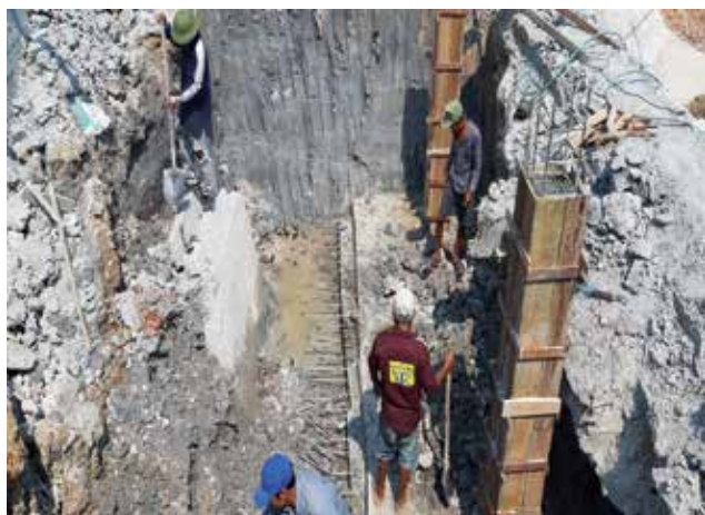
Raft Foundation for Pump House
