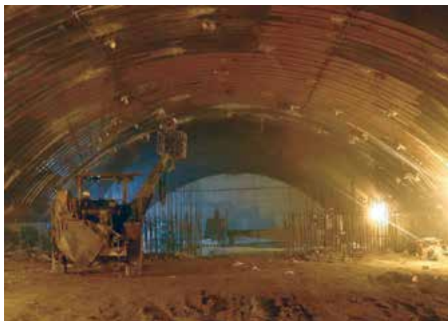
Strengthening measures and construction of RCC wall at DSG (South), Punatsangchhu-II
