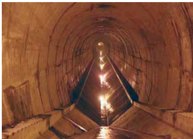
Desilting Chamber, Punatsangchhu-II, Hydro Electric Project
