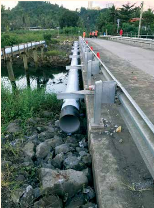
Anchor of pipe with bridge
