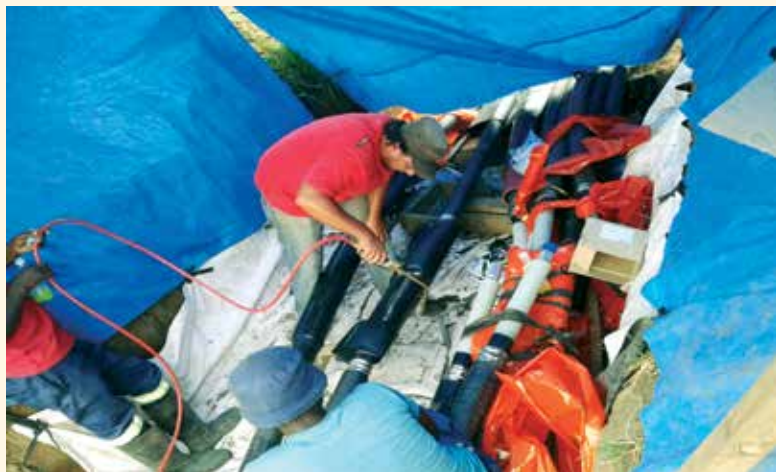
33kV End Termination Structure with LA at SE-2
