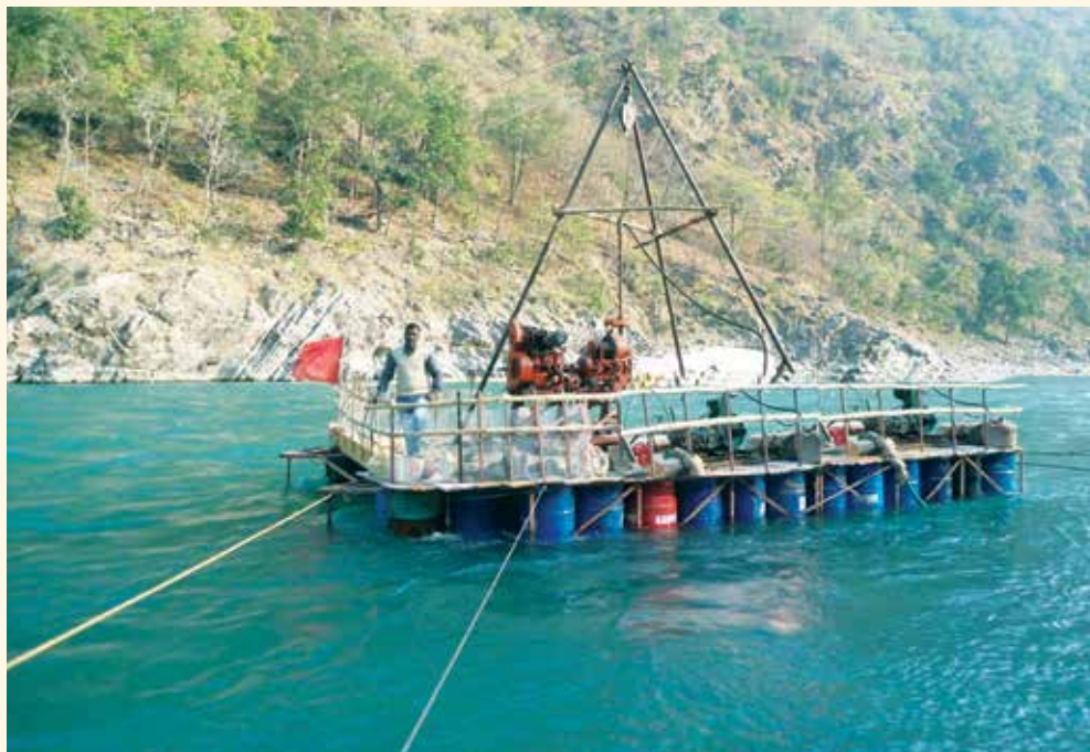
Under Water Drilling at Rupaligad Dam site
