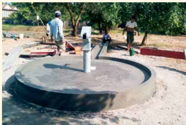
Installation of Hand Pumps in Memot District of Kamong Cham Province
