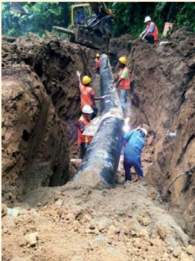
Laying of Waimanu Programme-2 works pipe - Welding on Bend
