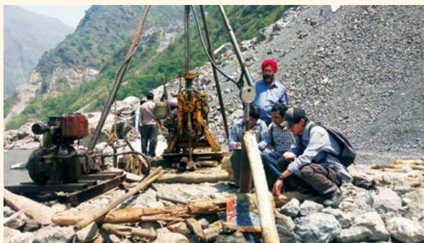
Core Drilling work at the Site Kuri Gongri H.E. Project
