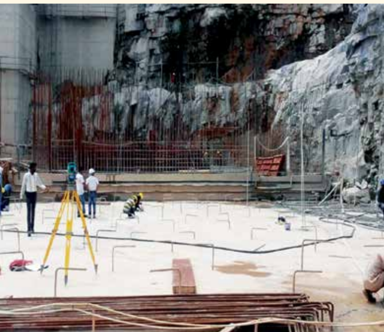
Marking of power house unit - II for Grand Katende Hydro Electric Project
