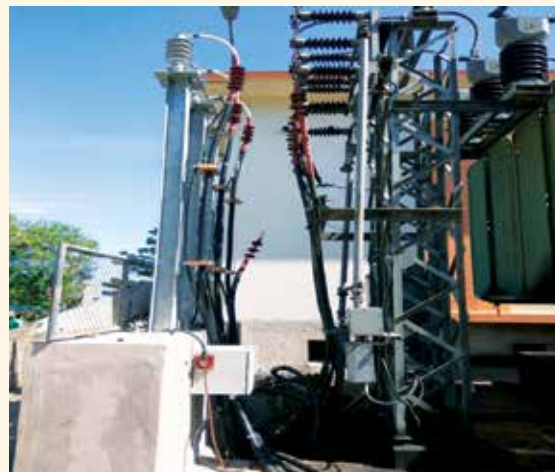
66kV Cable Jointing in CFM
