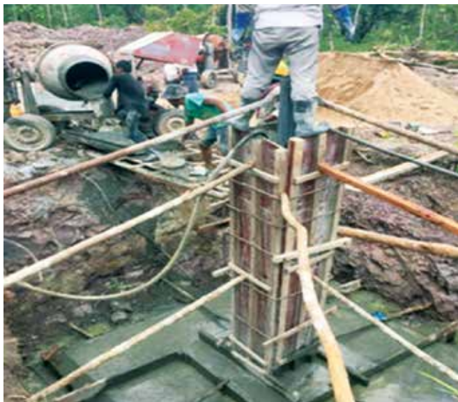
Foundation and casting activities at Project Site of 230kV D/C transmission line project from Stung Trengto Kratie, Cambodia
