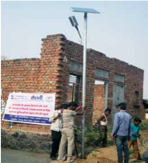
Installation of Solar Street Light in a village of Alwar, Rajasthan
