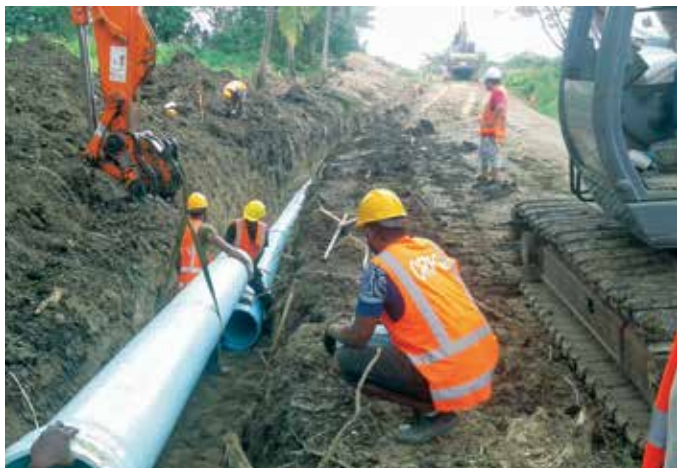
Joining of DN 375 Pipeline under WAPCOS supervision at Delaisiro, Fiji
