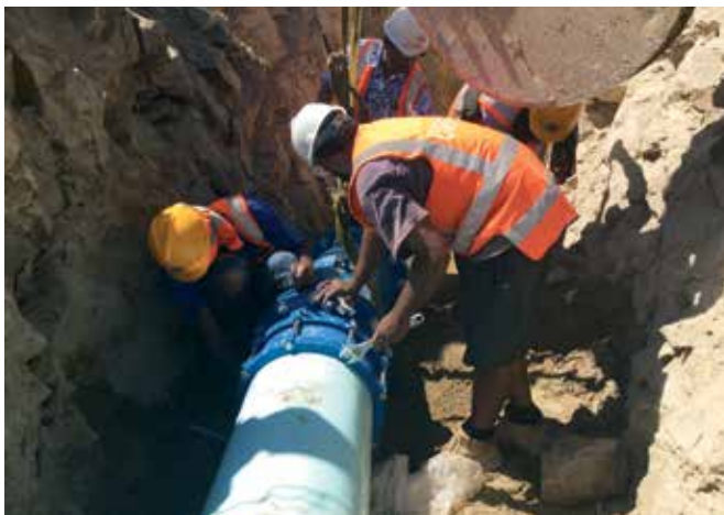
Installation of bends of DN 375 Pipeline under WAPCOS supervision at Delaisiro site, Fiji
