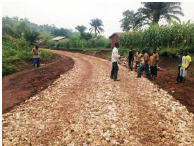
Stone pitching works for access Road, Kabu-16 HEP project, Burundi
