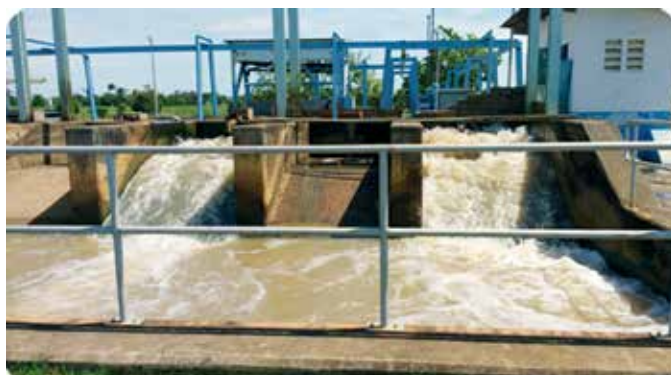
Intake structure at upper rivu, Water Supply Scheme in Dar Es Salaam and Chalinze, Tanzania
