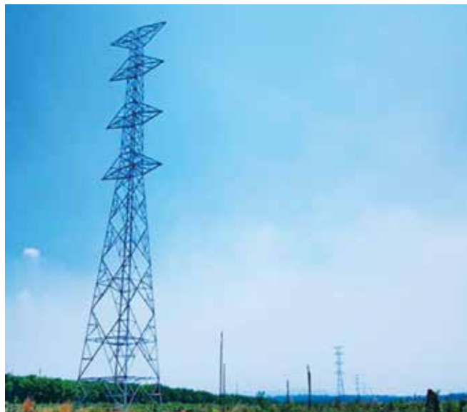
Transmission Line Tower (Suspension – Da Type) at Angle Point - 3/4 Along the Transmission Line Route, Stung Trengto Kratie, Cambodia
