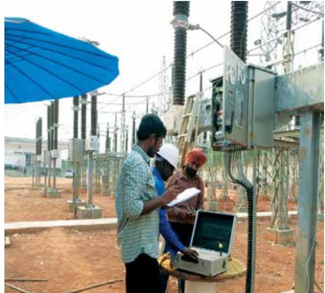
Pre-commissioning test on one of the Circuit breaker in Nabong substation, Lao PDR
