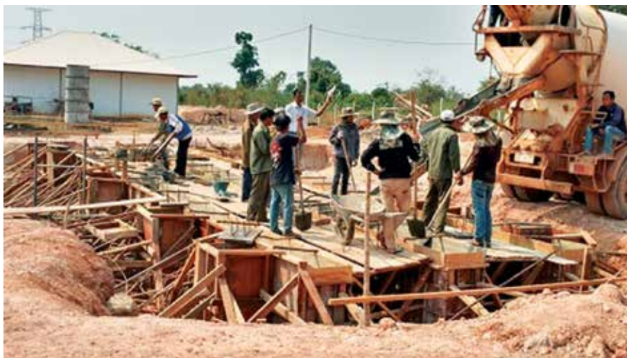
Casting of rail wall of Transformer foundation (No. 2) upto insert plate level in 230kV Nabong substation, Lao PDR
