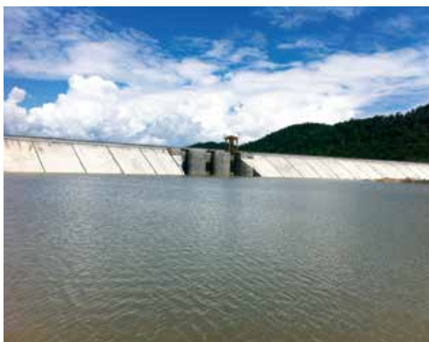
Stung Tasal Dam, a Concrete Faced Rockfill Dam is first of its kind in Cambodia built by state of the art technical expertise of WAPCOS, as Project Developer, under dispersive soil conditions in the region
