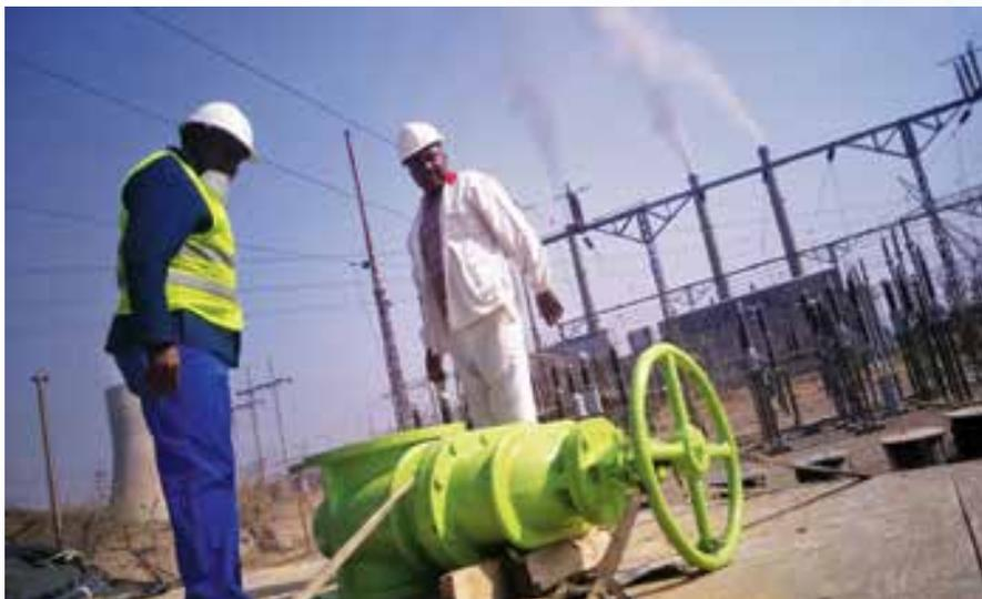
*Inspection carried on refurbished valves for Deka pumping Station*
