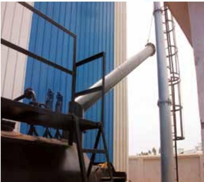
*View of Boiler Connection to Chimney, Fish Processing Plant*
