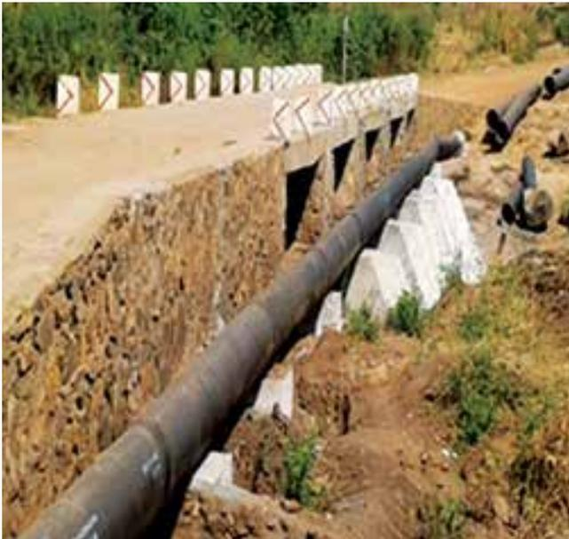
*Pipe Laying (Transmission Mains) at the Bridge crossing, Cuamba City Water Supply*
