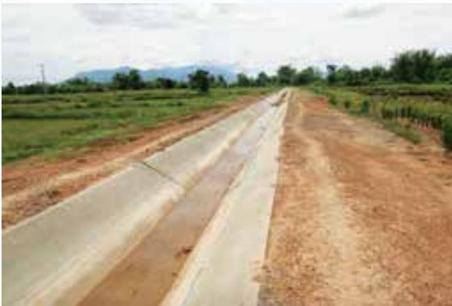
*Concrete lining work of Canal – Muang Sen Irrigation Scheme*
