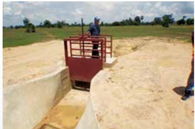
*New cross regulator installed at Muang Sen Irrigation Scheme*
