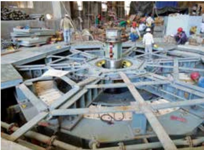
*Stator & Rotor in Place, Salma Dam Project*
