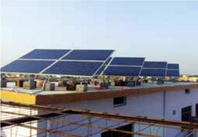
*Installed 5KW Roof Top Solar Power Generating System*
